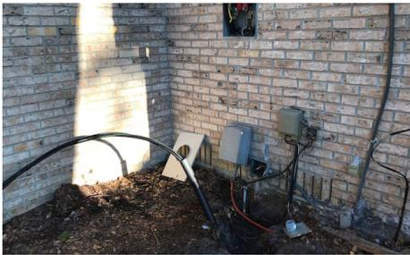
Every utility has to deal with temporary cables that are installed above ground because an underground cable has failed. These provi-
